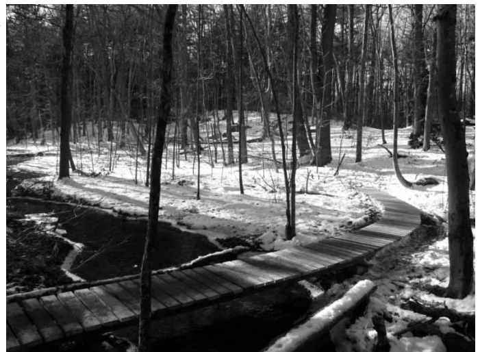
New 65 foot bridge and boardwalk on the Cobb property
